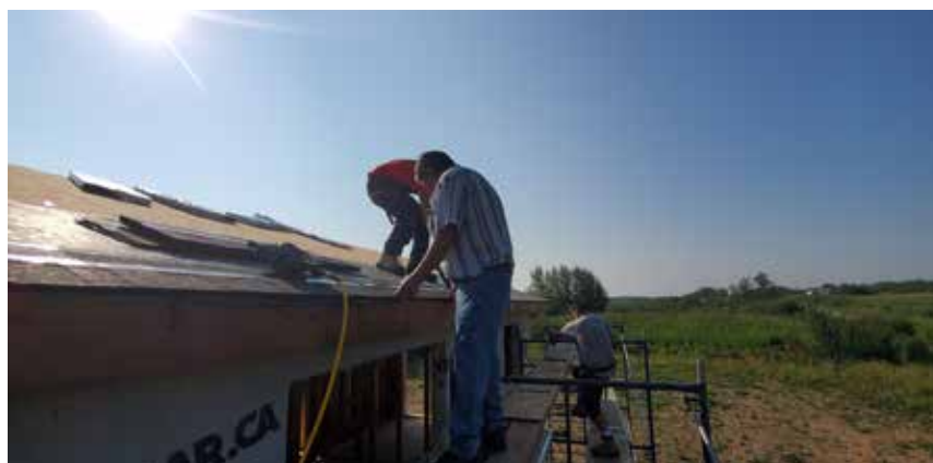
- The shingles of the "tiny home" being meticulously installed.
