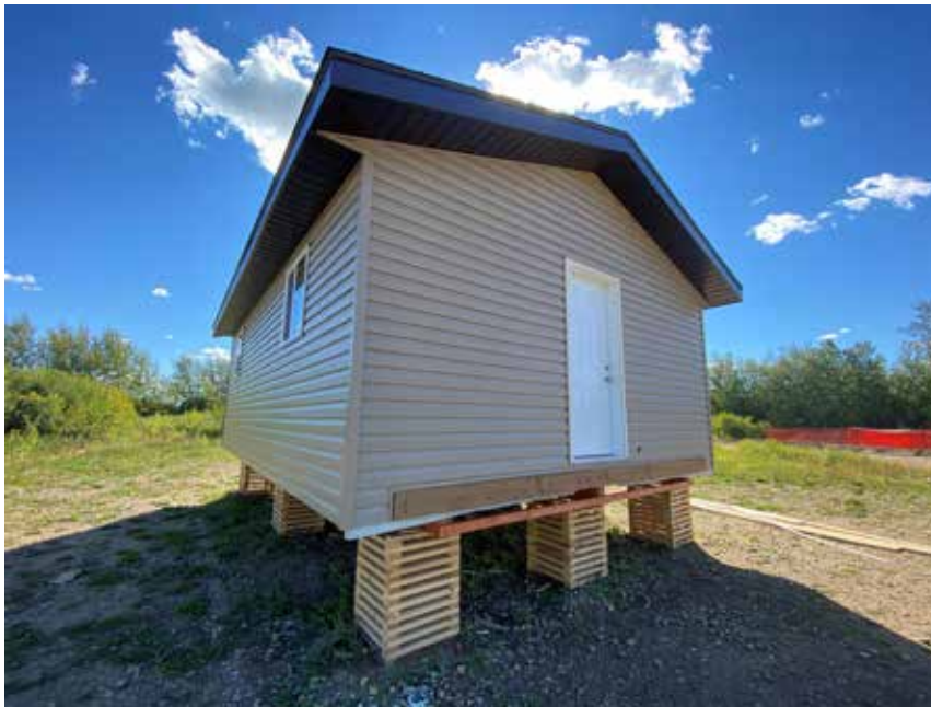
- The completed "tiny home" ready to be moved to it's final resting place.
