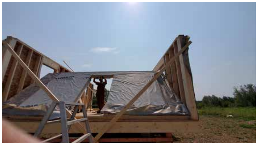
- Walls being raised into place.
